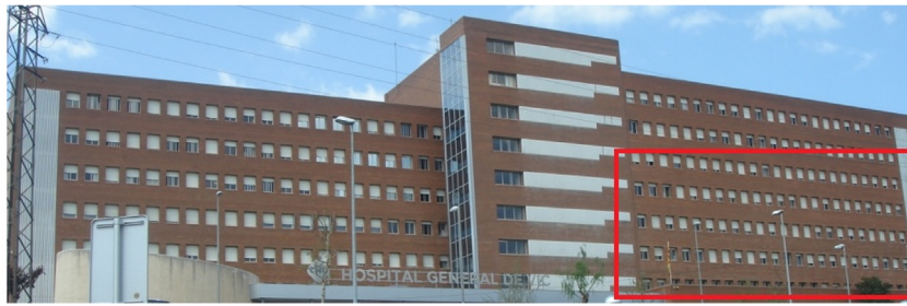
Fig. 1. Hospital section where the monitoring system was installed.
